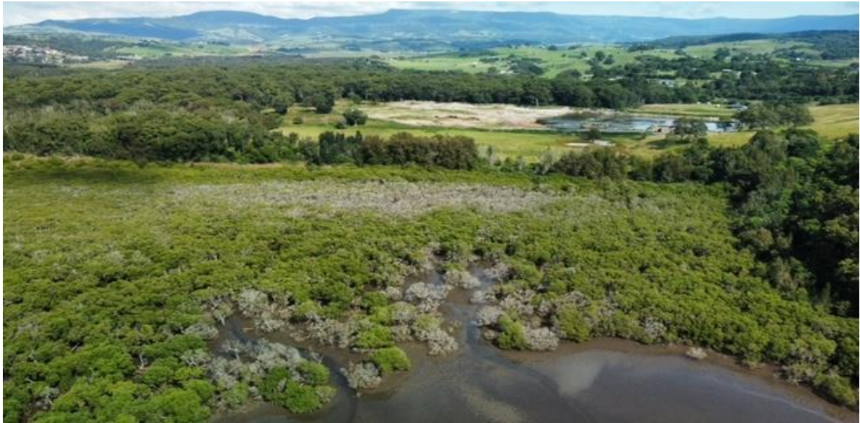
FOMR Photo 1 – 16-04-24: An overview of the main areas of dieback in the Minnamurra River estuary ecosystem: Boral Limited's Site 5B dredge pit, dredge lake and surrounding earthworks in its leasehold area is at top, about 200m from the start of the estuary intertidal zone in which can be seen, at centre, the larg egrey dieback area extending nearly the width of the Boral leasehold. The dieback is extending generally easwards along tidal channels to a further dieback area, the grey areas at bottom, closer to the river's main channel.
