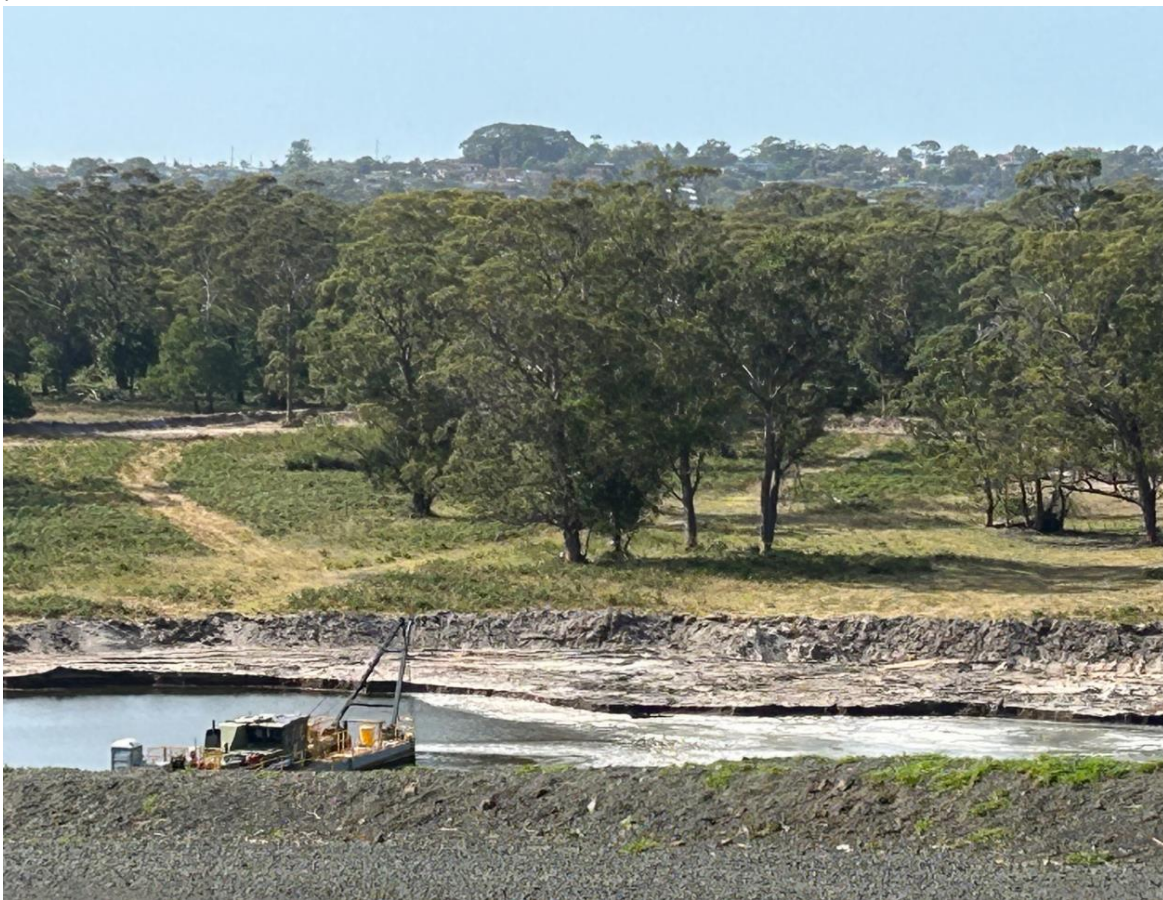
FOMR Photo, 30 October 2023: Boral Limited sand mining under way on its Site 5B, Dunmore/Minnamurra, the likely massacre victims' burial site and an area of highly protected ecosystems whose legislated protections the NSW and Federal governments are allowing to be overridden.
